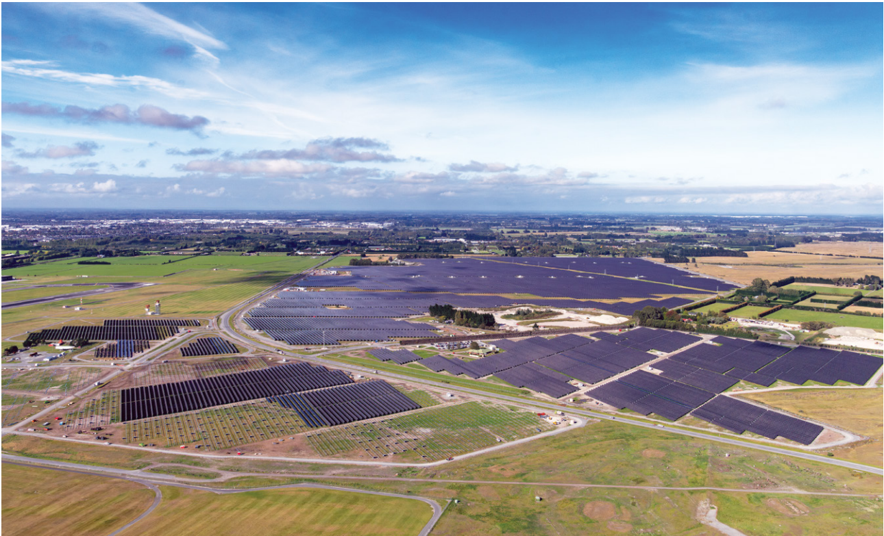
Christchurch International Airport's Kōwhai Park, one of the biggest solar farms in New Zealand, ready for commissioning.
